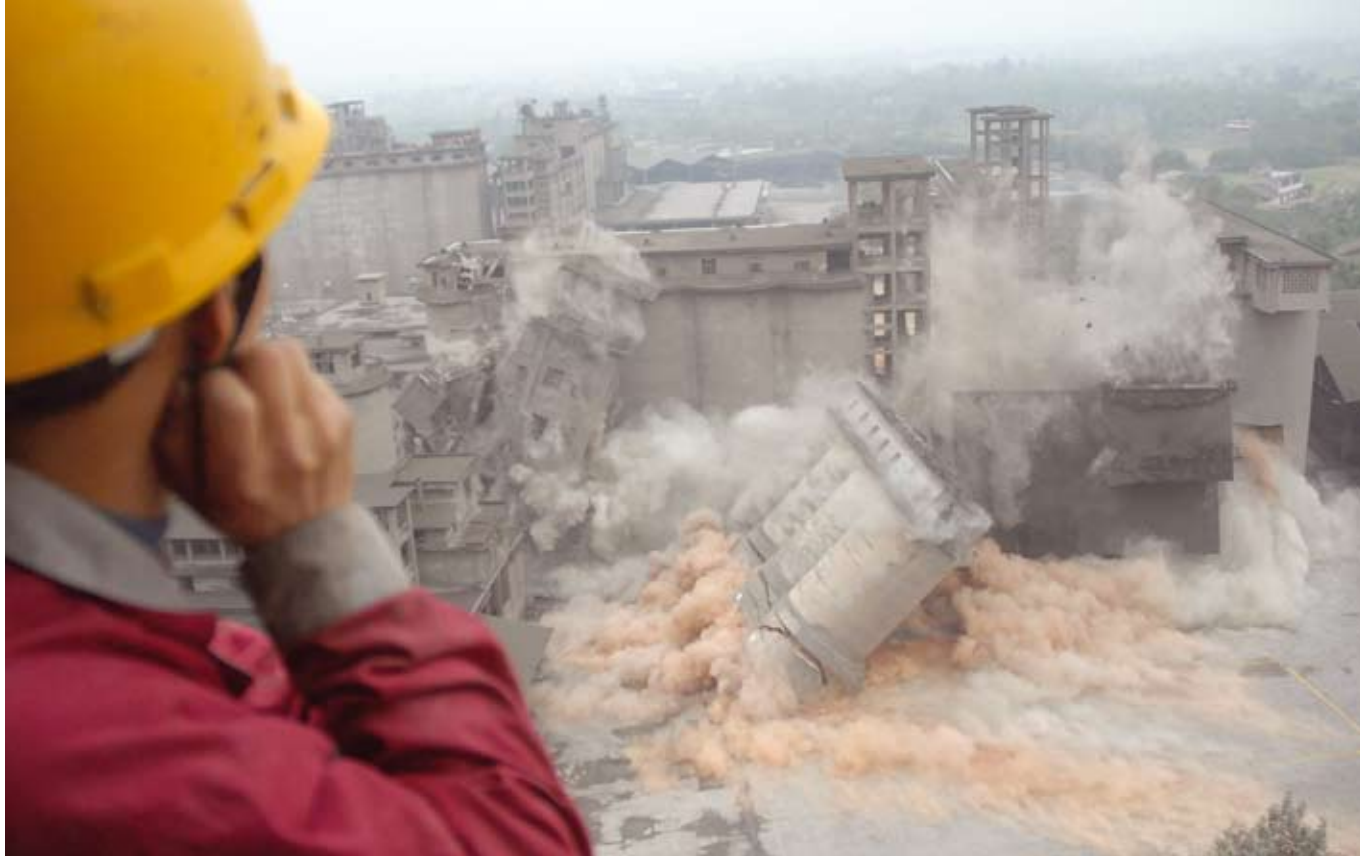
A heavily polluting cement plant is demolished in China's Sichuan Province. REUTERS/China Daily
