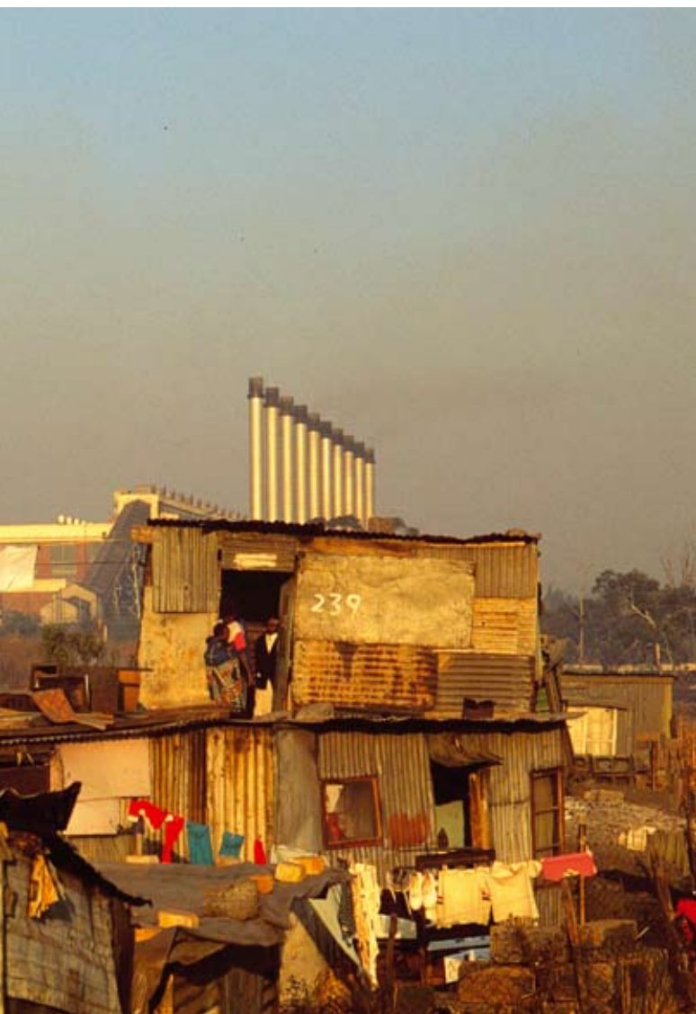
A squatter camp and high-tech power station in Soweto ... SA has a relatively well-developed economy, but lacks the social cohesion needed for a developmental state. Henner Frankenfeld/PictureNET Africa
